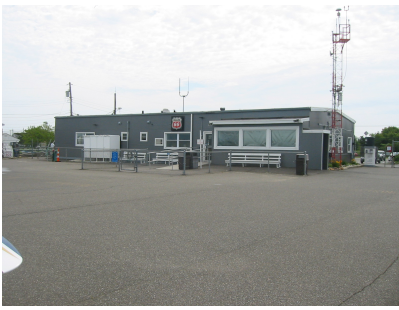
Entrance from ramp
